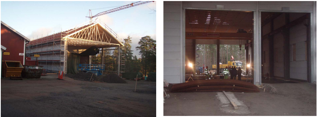
Figure 3-1 Bentonite Laboratory under construction.
